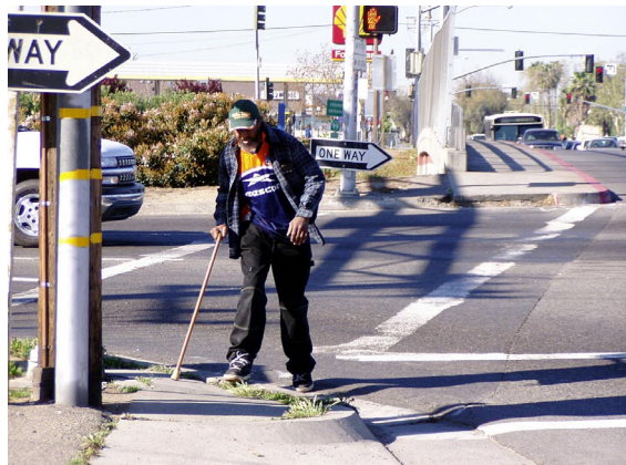
Many West Fresno intersections lack curb cuts. Signals should be timed to allow people with limited mobility adequate time to cross.
