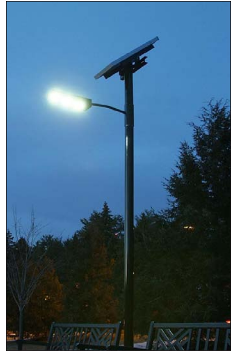
Above: An example of a solar street lights that could provide a safer environment for pedestrians without putting stress on the existing electrical grid.
