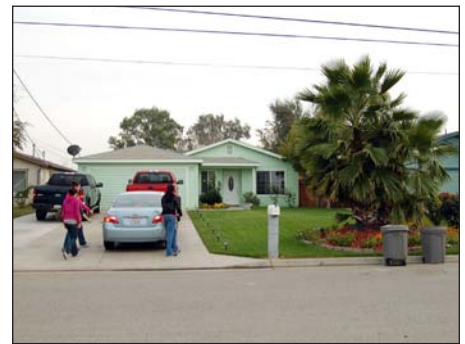
Above (from top to bottom): Vacant shell of the old Mammoth Orange Hamburger Stand along Highway 99; A well-maintained house and yard along Arnott Drive.
