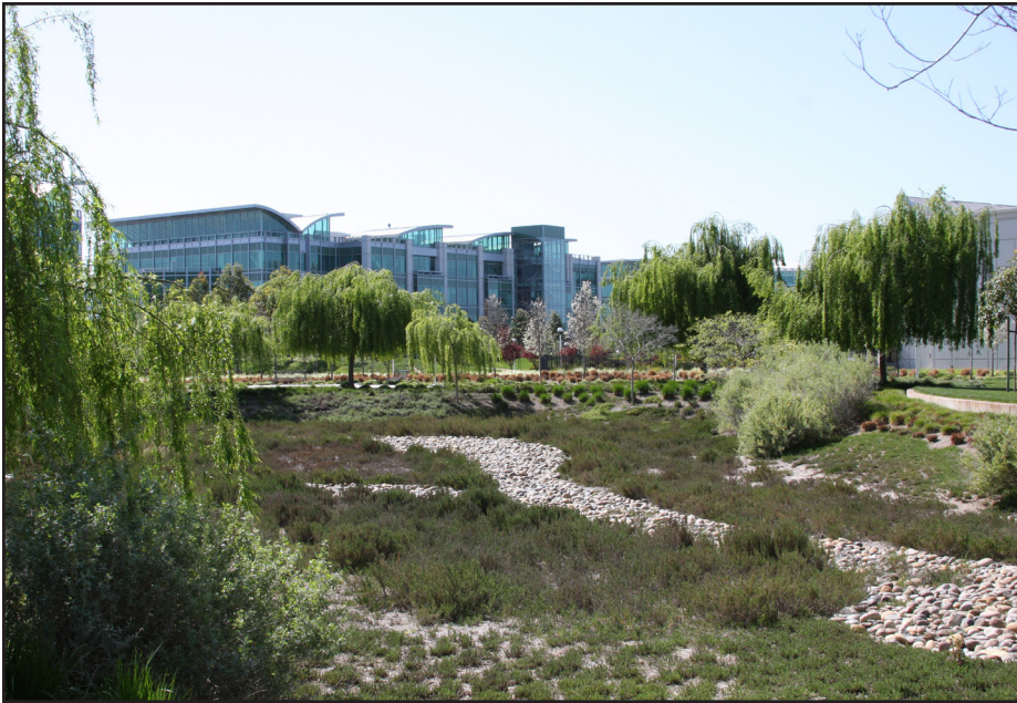
Storm Drain System Enhancement
