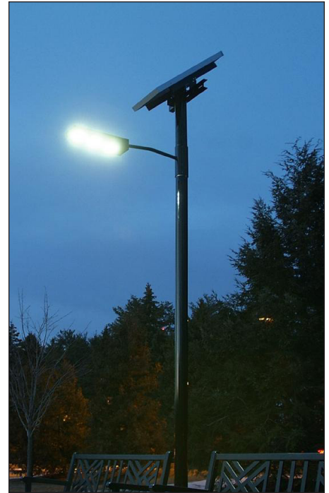
Above: An example of a solar street lights that could provide a safer environment for pedestrians without putting stress on the existing electrical grid.
