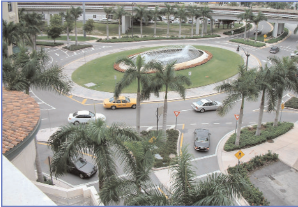
Dual-lane gateway roundabout in Coral Gables, FL.
