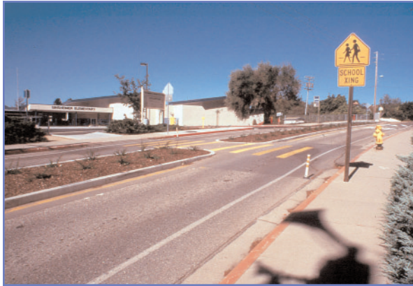
This speed table, or raised crosswalk, looks similar to the speed humps currently installed on McGirk Ave., but the top is flat with ramps. Drivers slow before reaching the speed table, which makes it an ideal local for a crosswalk.
