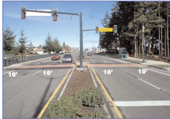
Reducing lane widths to 10 feet can provide space for bike lanes and medians. Note the improved pedestrian crossing.
