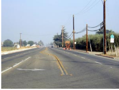
SR 63 (Road 128) looking toward Orosi at the intersection of Avenue 408 is typical of a suburban highway section that transitions to an urban highway. Even though this is a very short section of road, motorists feel comfortable driving fast here. Note the new sidewalk on the left side of the highway. There is no sidewalk on the right side of the highway, and no marked crosswalk in the vicinity.
