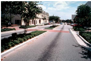
The bulb out and median in the photo above depict the type of design recommended on Avenue 416. The median provides a refuge for people crossing, whether at the school or near shopping. Crossing distance is greatly reduced by the median, the reduction in lanes, and the bulb out. Stop lines in advance of the crosswalk should also be used.
