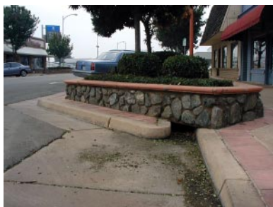
Tree wells, like the one shown above, can serve as an effective substitute for continuous planter strips.
