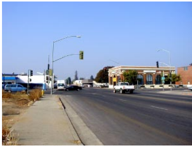
Existing conditions at SR 63 and Avenue 416.
