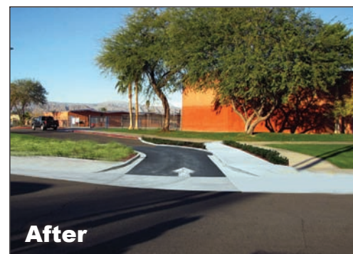
Figures 4.35 and 4.36: Photo simulation of a narrowed entry point for student dropoff/pickup at Cesar Chavez Elementary. (This improvement would need to be constructed by the school.)
