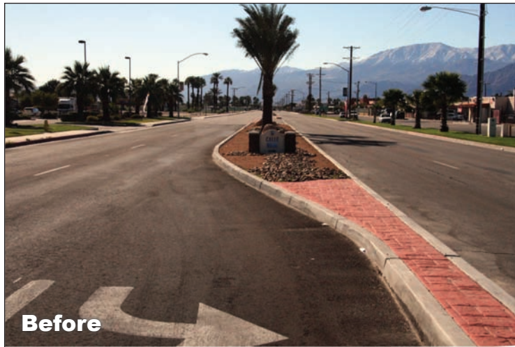
Figure 4.1: Harrison Street as it is today.
