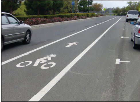
On this street, they have created a 4 foot buffer between the parking aisle and the bike lane to use up more of the excess width.
