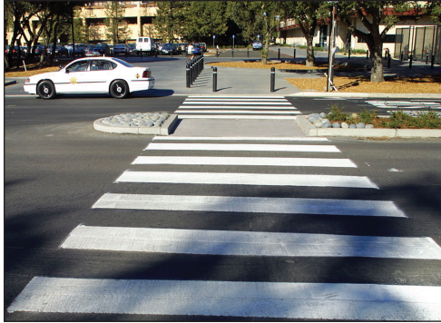
Example of crosswalk through median with a median nose to provide shelter for pedestrians.
