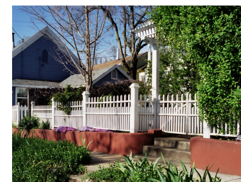
Wood fence is raised on a low masonry wall
