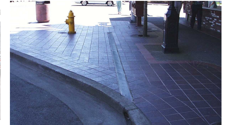
A permanent curb extension
