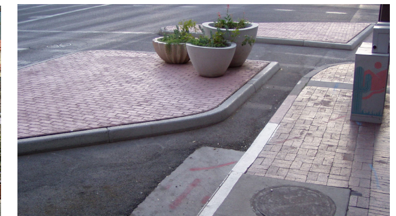
This curb extension allows water to drain to the sewer inlet, following the existing drainage line.
