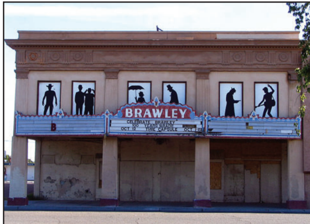
Potential opportunity for renovation.
