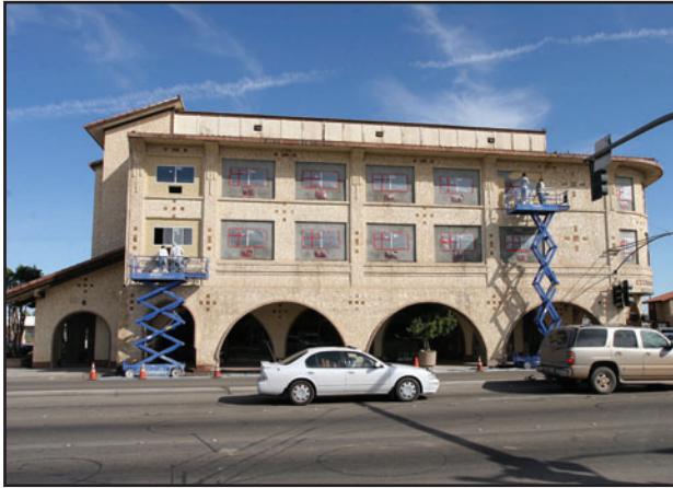
Current renovation in progress in Brawley.
