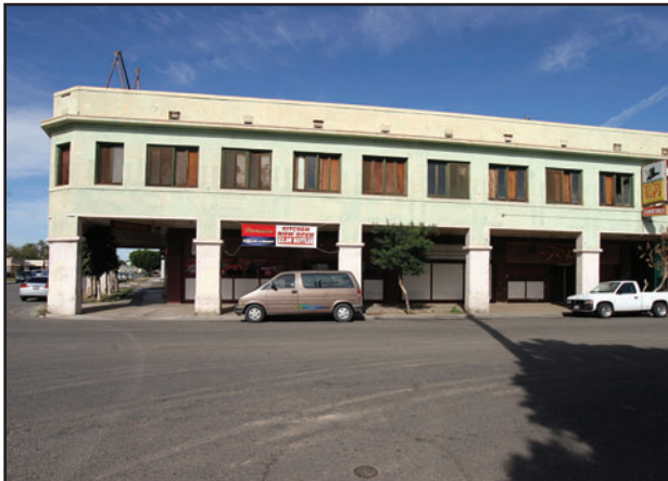
Another potential opportunity for renovation.
