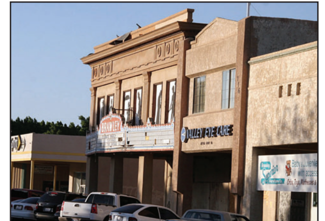
Old theater is a prime renovation opportunity.
