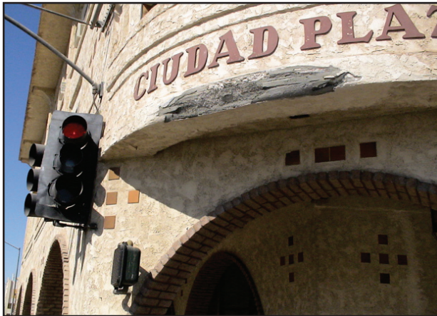
The Ciudad Plaza building is frequently damaged as large trucks negotiate the tight right turn onto Main Street.
