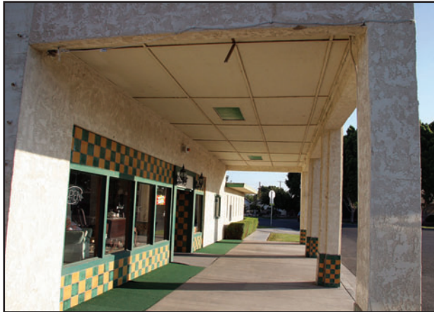
Plaza Park area commercial buildings.
