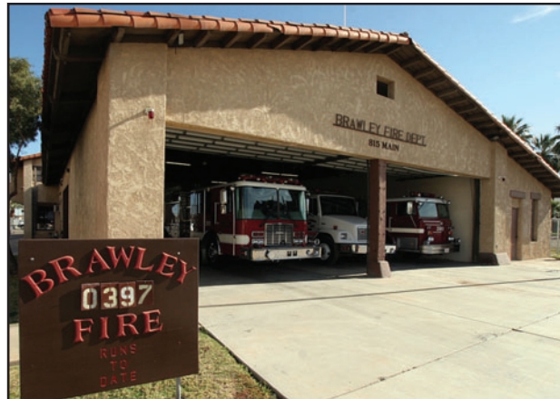
Brawley Fire Department headquarters.
