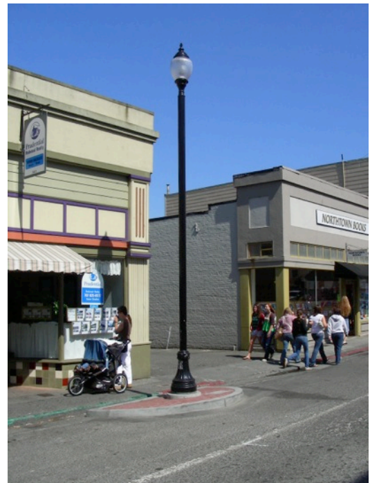
Curb Extension with Lamp
