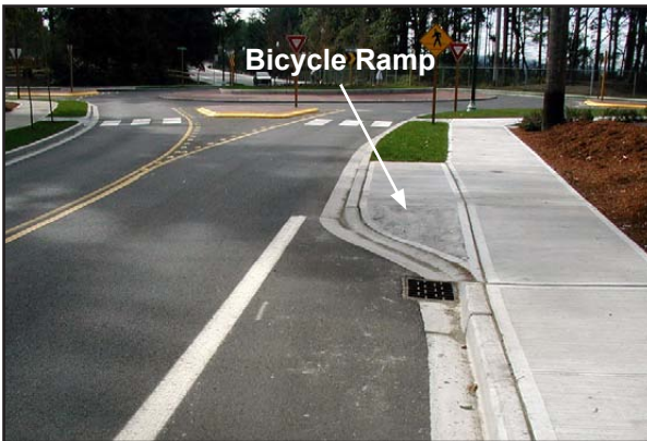
Ramp for bicyclists at roundabout.
