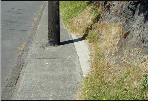
Example of sidewalk widening around existing utility pole.
