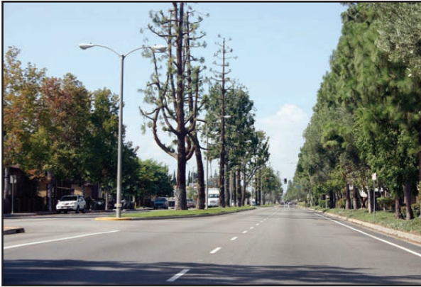
Missing sidewalks and too-narrow bicycle lanes.
