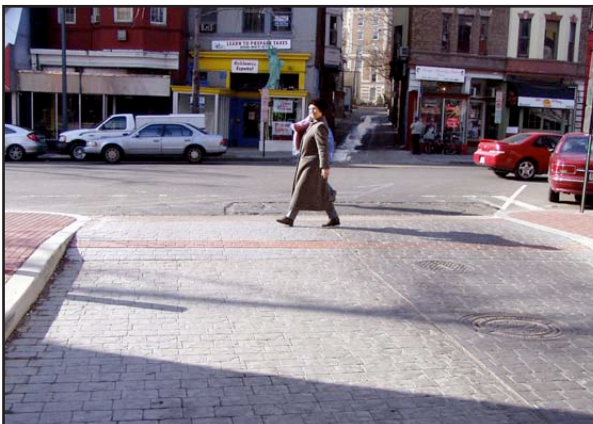
Raised crosswalks across streets and driveways provide a continuous, level path of travel for pedestrians.
