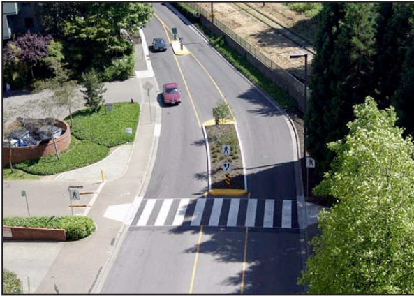
High-visibility, ladder-style crosswalk.
