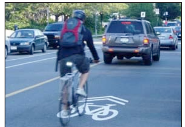
This “sharrow” on a Class III bicycle facility helps drivers and cyclists alike know how to use the roadway safely.
