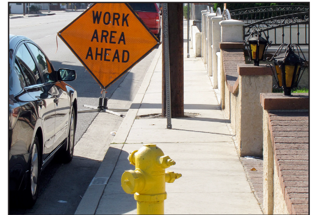
Narrow sidewalks, sometimes with barriers.
