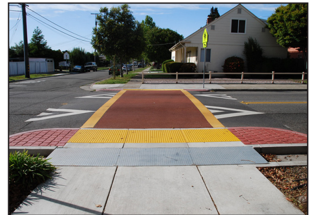
The two above photos show a speed table in front of a school from different views.
