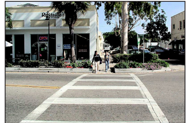
Intersection with bulbouts, two pedestrian ramps, and high visibility crosswalk.
