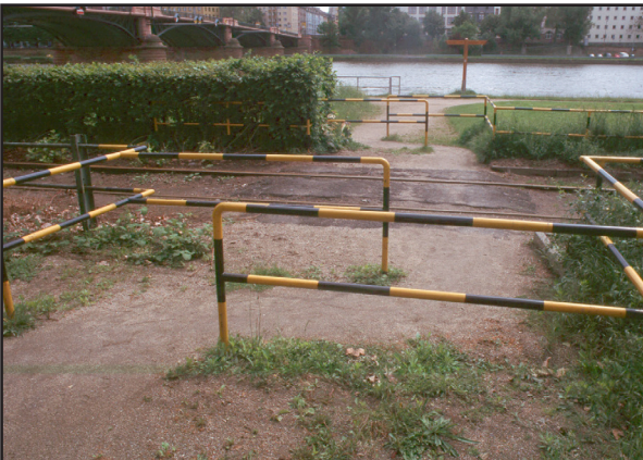
Example of S-shaped element by railroad tracks. The directional changes force pedestrians to look in the direction of the train before crossing.
