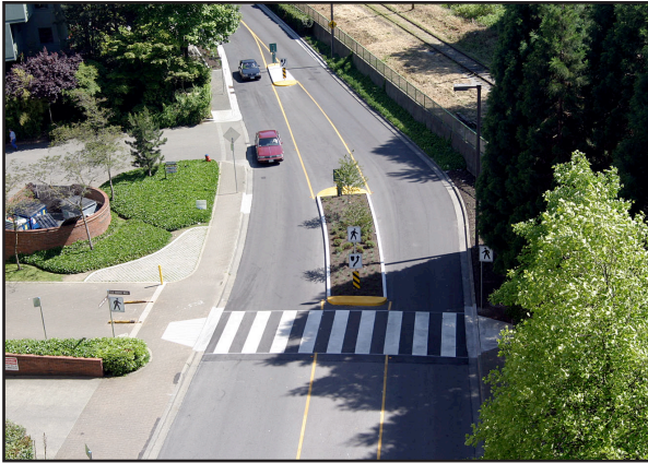
High-visibility, ladder-style crosswalk.
