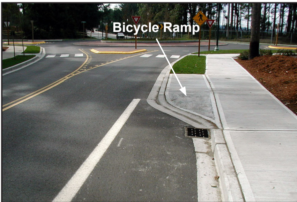
Ramp for bicyclists at roundabout.
