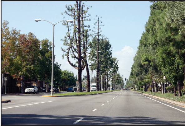
Missing sidewalks and too-narrow bicycle lanes.
