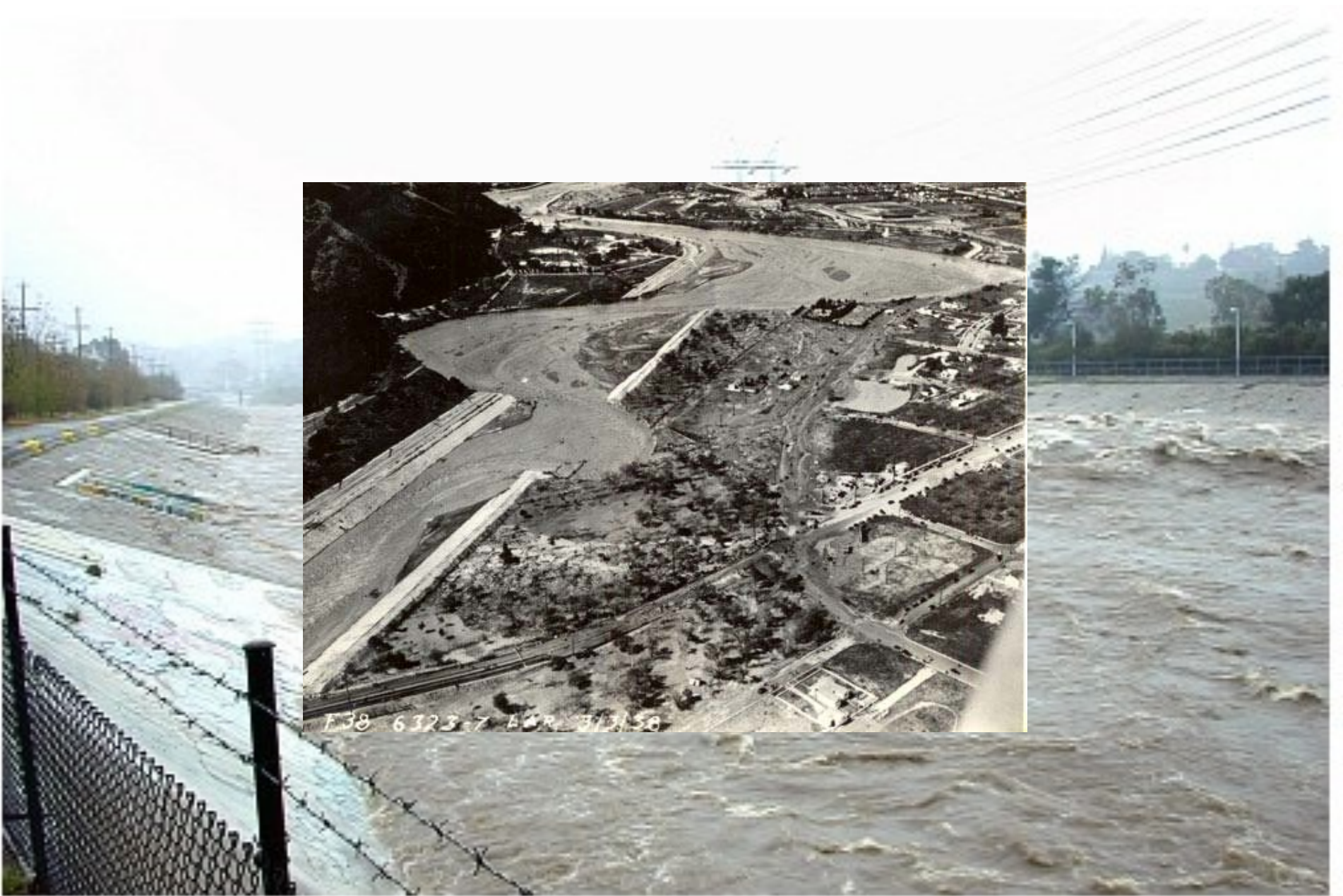
Los Angeles River near Victory Boulevard, Feb-Mar 1938
