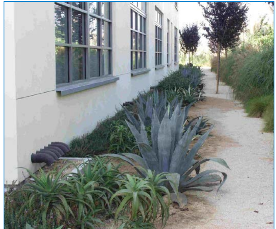
Roof drain into drywell
